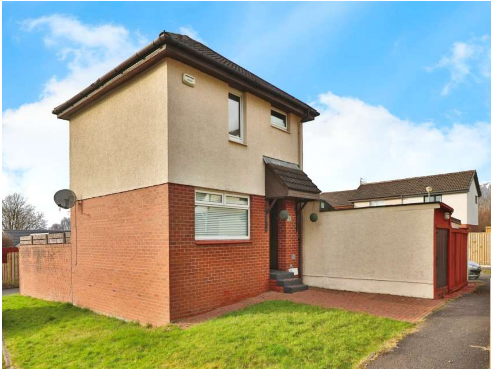
Auchinleck Crescent, GLASGOWG33 1PT
