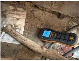
The top of floor joists to rear where accessible tested dry at time of survey
