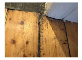
Signs of common furniture beetle attack in sanded and sealed floor timbers
